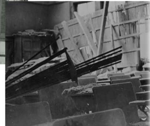
Courtenay Elementary School
